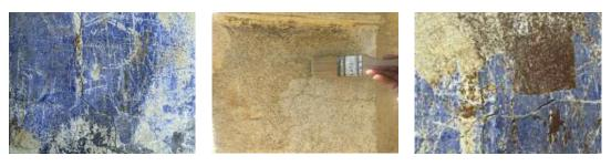
The structure presented problems of a static nature. Also, the plasters and the painted surface were extremely degraded and uneven. In fact, the weathering had caused loss and detachment of plaster and had washed the layers of paint.
