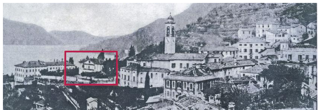
Marked in red, the building that was the first seat of the kindergarten, today's Town Hall
